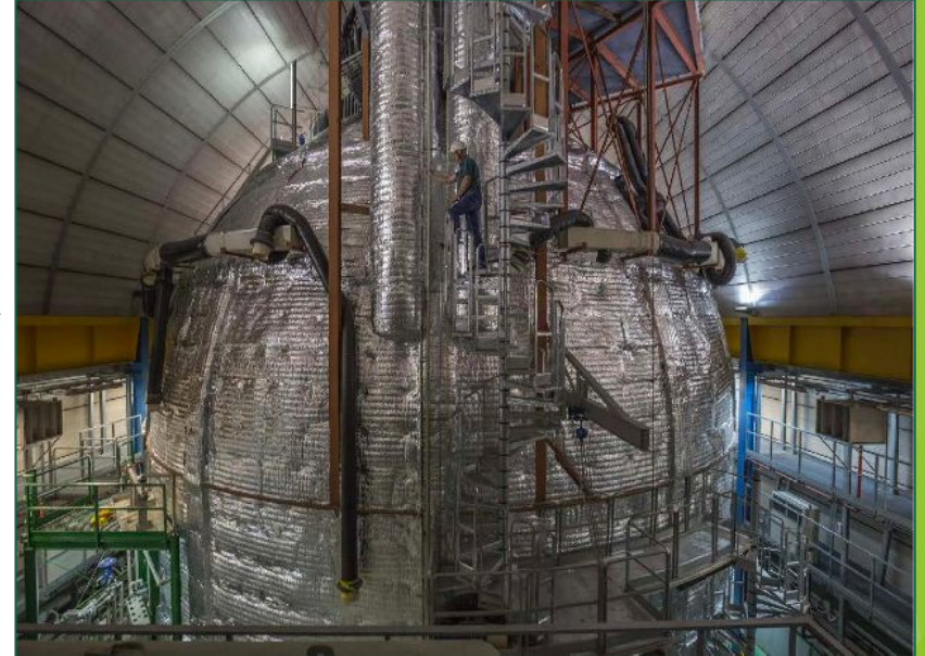
After the thermal insulation (Early 2016)
